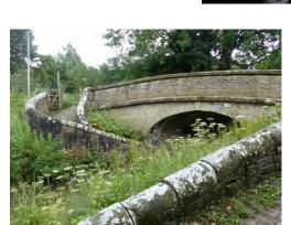
Bridge 29 is a roving bridge. These bridges, a speciality of the Macclesfield Canal, occur where the towpath changes sides, the spiral ramp allowing the towing horse to switch from one bank to the other without having to be unhitched from the boat.
