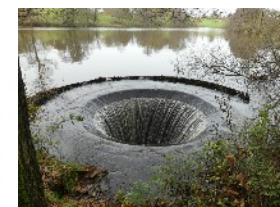
The ornamental lake at North Rode Manor hosts waterfowl including Cormorants, Teal, Mandarin Ducks and Goosanders. The lake's outflow departs via this distinctive shaft spillway.
