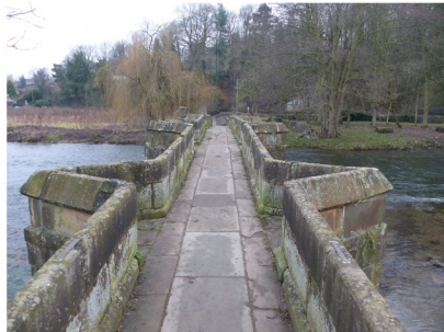
Holme Bridge is a fine example of a packhorse bridge, spanning the River Wye above Bakewell. It dates from 1664 and is a Grade I listed building. Packhorse bridges offer a reminder of the days before canals, railways and lorries, when bulky goods such as salt were carried by trains of pack ponies on long-established routes across the country. Packhorse bridges are typically narrow, with low parapets (or none at all) to avoid fouling the panniers carried by the laden animals. Many, as here, have triangular pedestrian refuges extending above the cutwaters between the spans.
