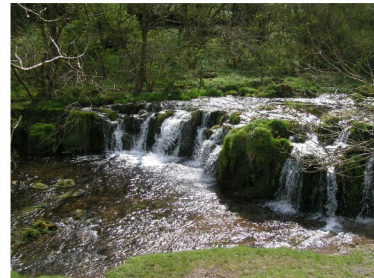
Despite its natural appearance, the Tufa Dam is thought to have been built by fishermen in the 1930s. Tufa is a porous rock created when dissolved calcium carbonate in lime-rich water is deposited on moss.
