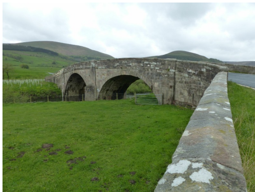
Burholme Bridge carries the road over the River Hodder. It was built of sandstone ashlar in the late 18th century and is Grade II listed.
