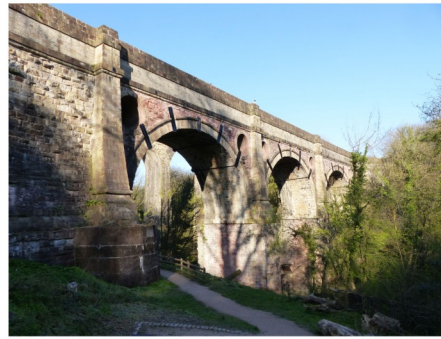
Marple Aqueduct , carrying the Peak Forest Canal over the River Goyt, is the highest canal aqueduct in England, and the highest masonry-arch aqueduct anywhere in Britain. It was designed by Benjamin Outram and opened in 1800.
