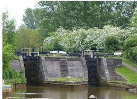
Many of the Trent & Mersey Canal locks are doubled; the long flight east of Wheelock is nicknamed "Heartbreak Hill". The canal runs from the Trent in Derbyshire to the Bridge-water Canal near Runcorn, and thence to the Mersey.
